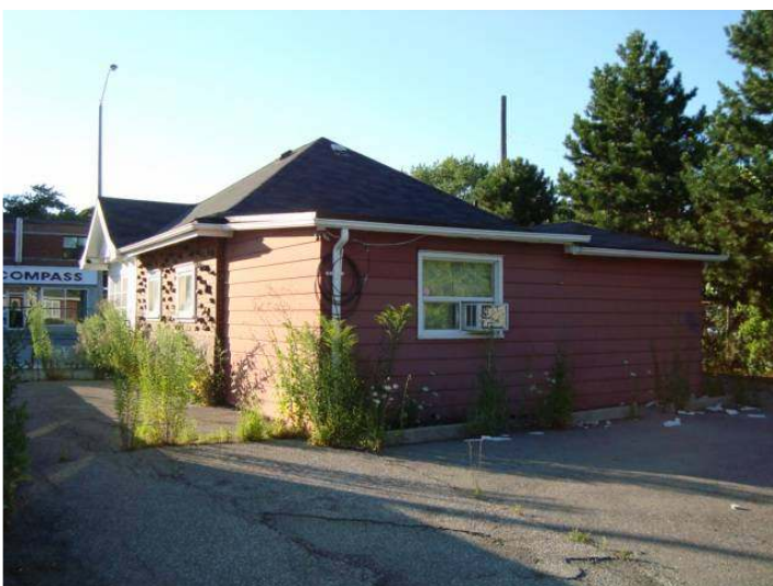
July 2010: Steel fencing harming the wooden exterior, graffiti, 2 broken windows, ripped screening, weed overgrowth, ease of access and damage to roofline.
