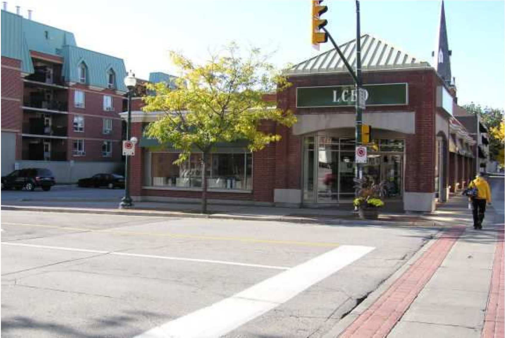
LCBO Store – former Esso service station
